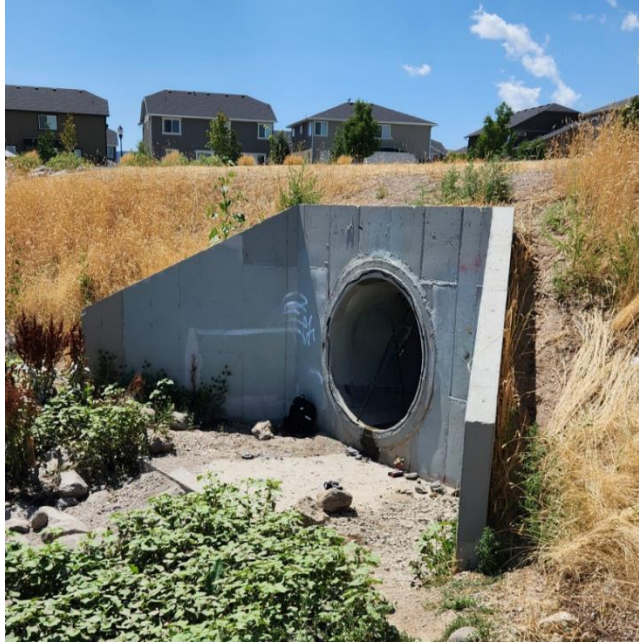
Figure 1. Culvert under a road
